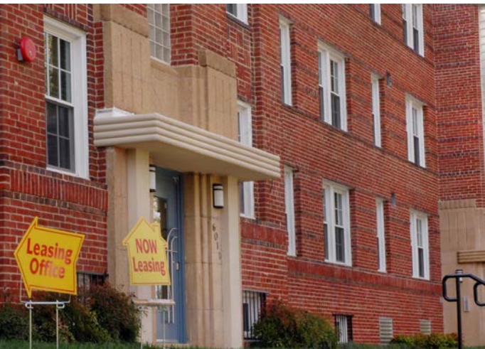
Fort View apartments, our 62-unit affordable housing property in Ward 4.
